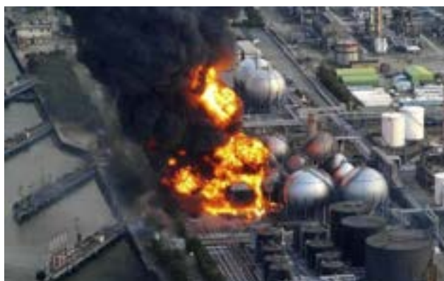
c) LPG tank farm at the Chiba refinery Japan after the earthquake,
