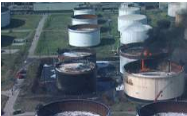
a) AKSA acrylic fibre plant disaster post Earthquake, Turkey, 1999
