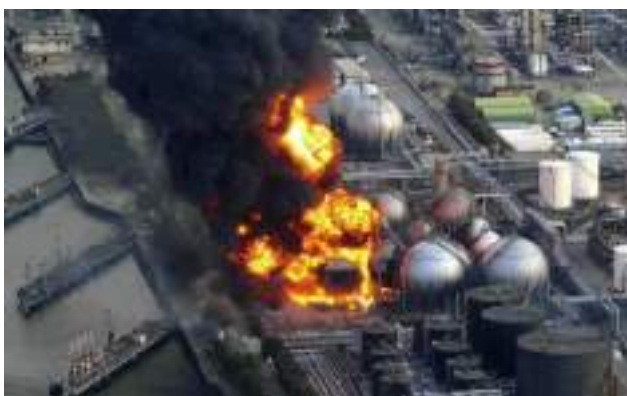
c) LPG tank fire at the Chiba refinery, Japan after the earthquake 2011
