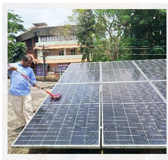
Figure 6: Cleaning of PV modules
