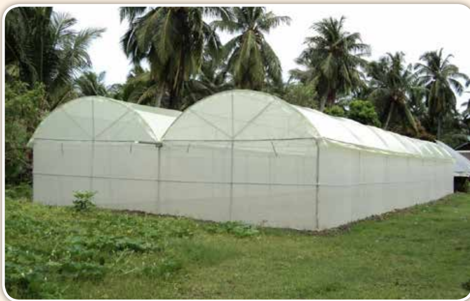
Construction of Hi-tech polyhouse
