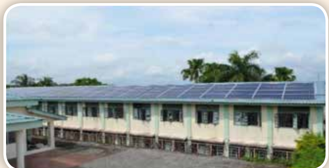
1 MW rooftop solar plant installed in 15 govt. buildings & 3.15 MW rooftop solar plant installed in South Andaman (33 buildings) & Car Nicobar (6 buildings).
