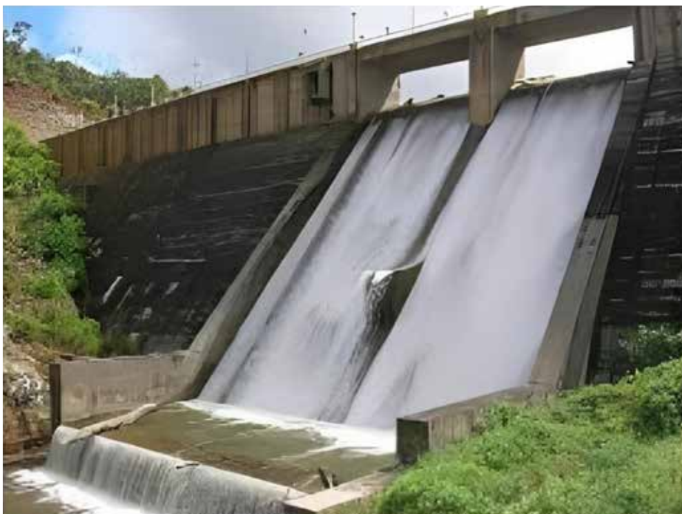
Kalpong Hydro-electric power project in North Andaman
