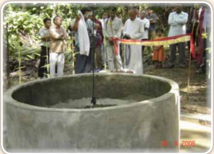
Construction of RCC Ring well under minor irrigation scheme
