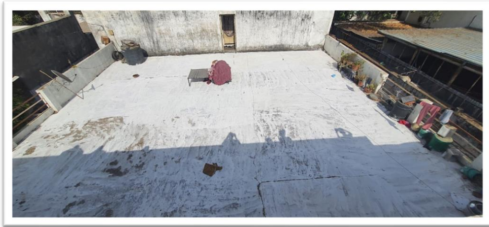
Image 8-9: White painted cool roof and visit to low-income houses that have adopted cool-roof measures, Shahibaugh, Ahmedabad
