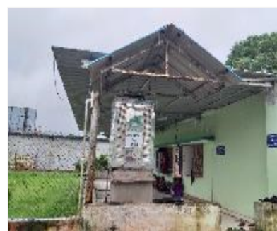
Figure 6: Solar operated water heater, CHC Bairamgarh
