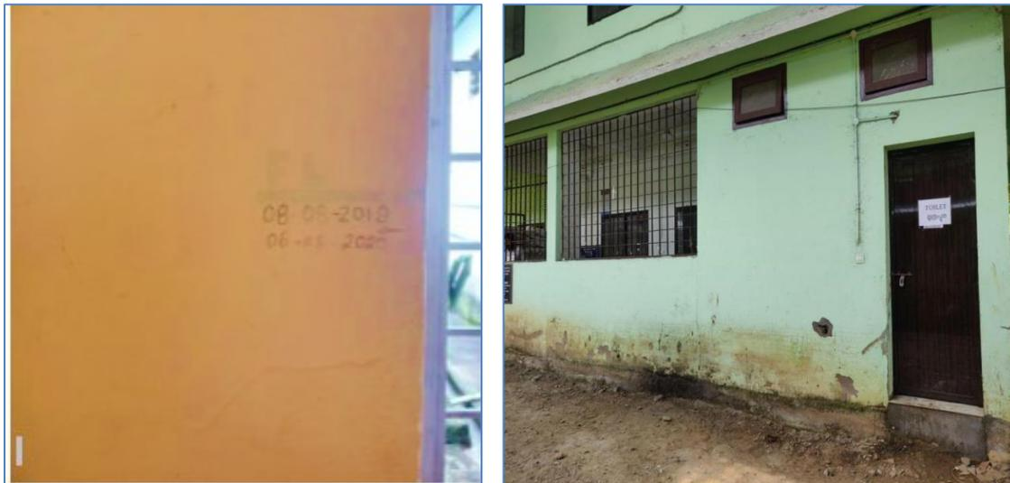
*(Left) Flood water levels marked on the wall, (Right) Dirt in walls due to flooding, Vandiperiyar CHC*
