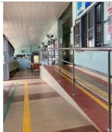
*Newly constructed PHC floor with higher floor level, high wall tiling and ramps, FHC Pozhuthana, Wayanad, Kerala*
