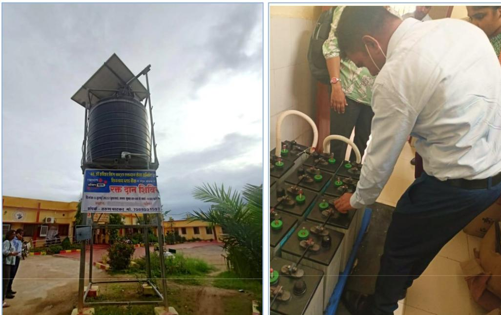
(Left) Water tank connected to Solar Panels (Right) batteries of solar placed in a separate room, Patewa PHC, Chhattisgarh
