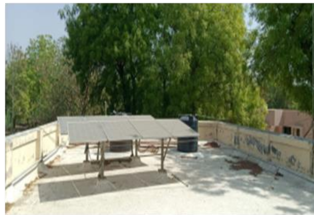
Tiled cool roof with solar panels in UPHC, Gujarat
