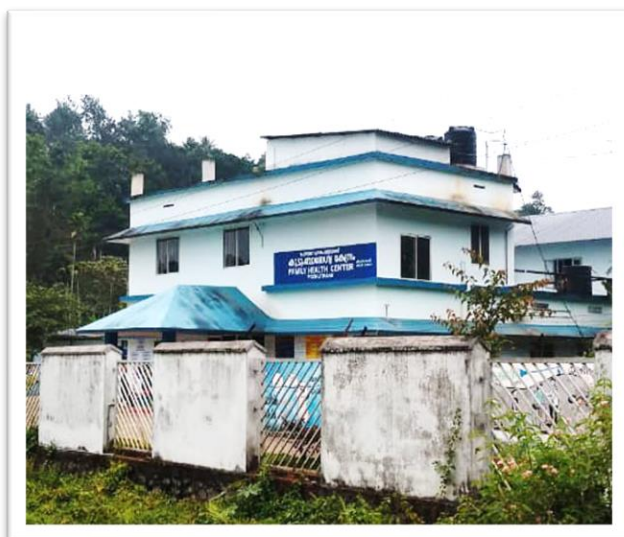
(Left) Compound wall of the PHC with metal grills. (Right) Ditch dug around the PHC building for easy drainage in case of floods and fenestrated walls with elevated waste disposal storage.
