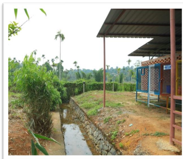
(Left) Compound wall of the PHC with metal grills. (Right) Ditch dug around the PHC building for easy drainage in case of floods and fenestrated walls with elevated waste disposal storage.
