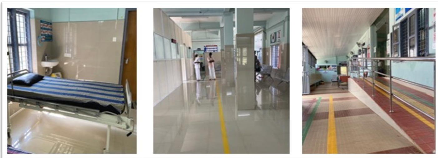
Tiled floors and elevated ramps to reduce impact of flood waters and ensure continued health care delivery, features of a flood-resilient health facility
